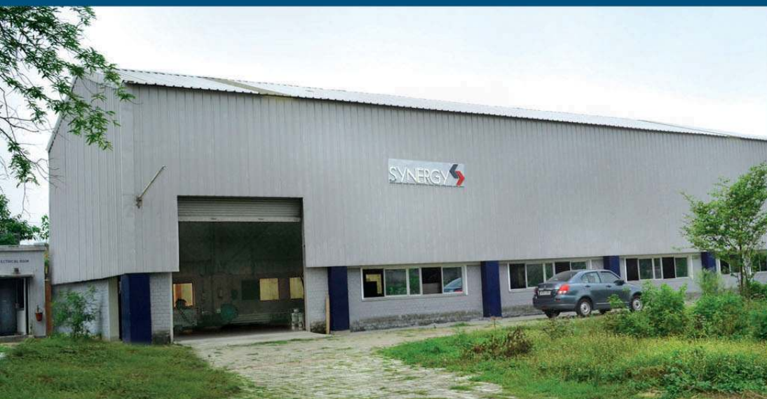
Synergy's Belt Vulcanizer plant at Kalyani, near Kolkata International Airport
